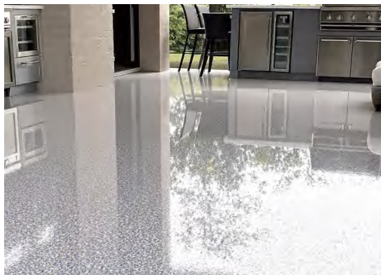
Epoxy Colored Sand Floor
